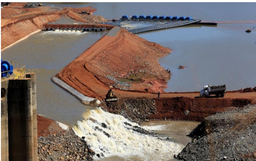
Figure 11. Floating pumps and cofferdam to tap Dead Storage
